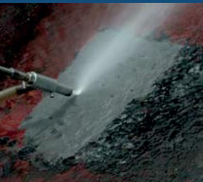
Wet Sand-blasting on Corroded steel plates
